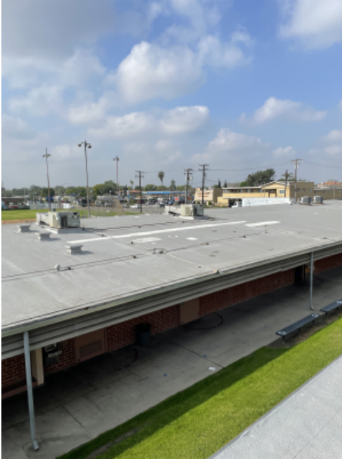
Building G Roofing Mastics (Patch, Penetration, Sleeper)
