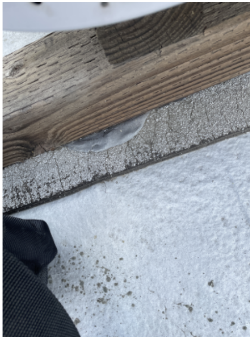
Building F Roofing Mastics (Patch, Penetration, Sleeper)
