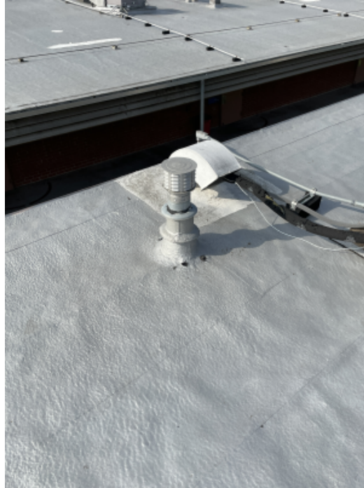
Building D Roofing Mastics (Patch, Penetration, Sleeper)
