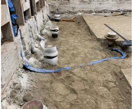
All the plumbing is complete in the interior and concrete is being finalized for both interior and exterior scope by early August. The project is roughly 70% complete. Wall framing, tile and restroom accessory installations are next.
