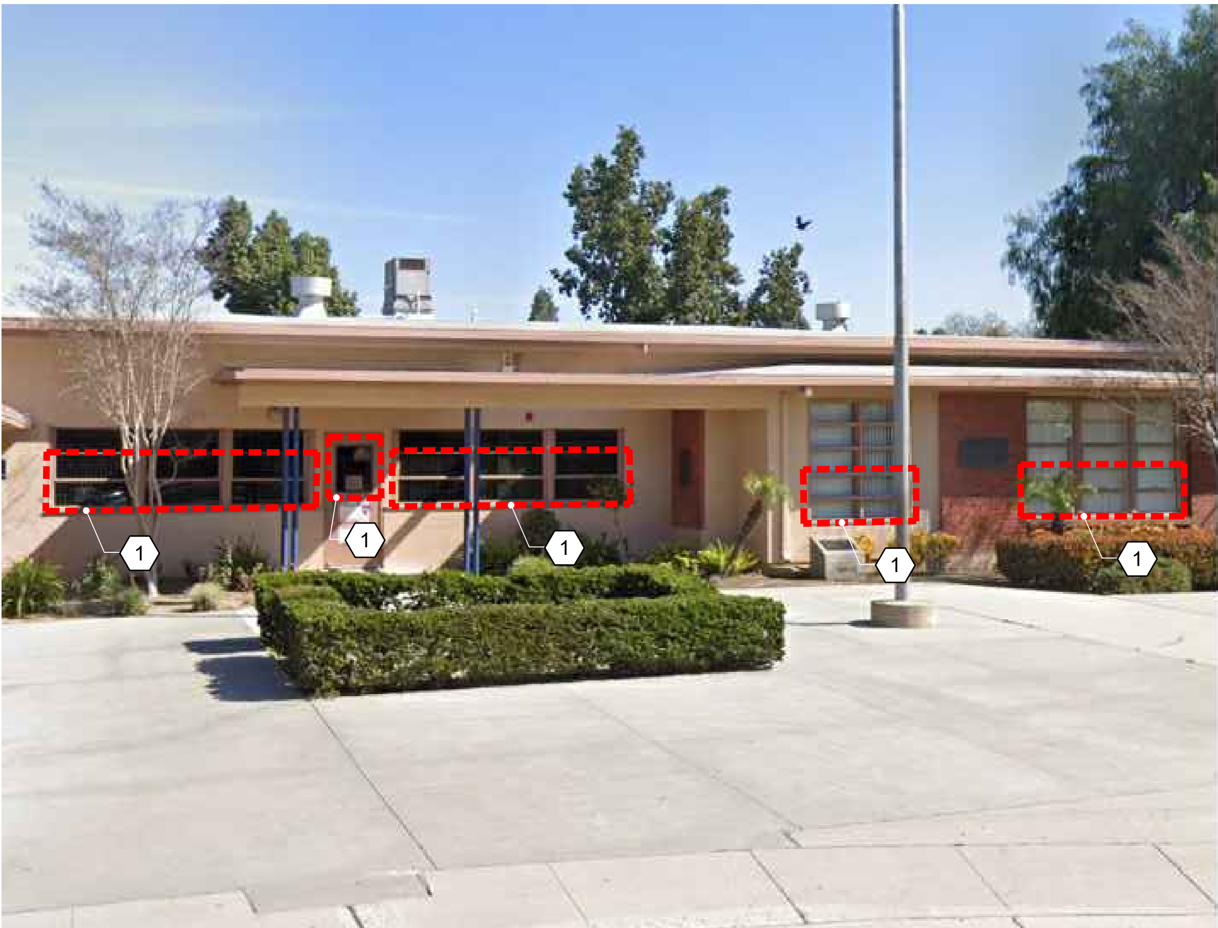
WARD ELEMENTARY SCHOOL
