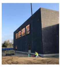
The new gymnasium is moving along and progressing as scheduled. The masonry contractors completed the block wall for the gym building. Structural steel contractors installed the high truss system.
