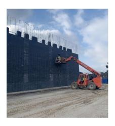
The masonry contractors are continuing to stack the black block walls while the concrete contractors are forming columns and lintel. School staff members were welcomed onto the construction site last month to sign the steel trusses.
