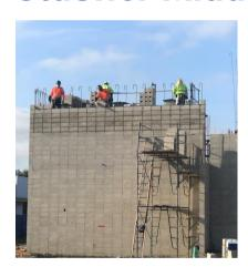
The masonry contractor is continuing to stack the block walls for the gym while the concrete contractor is working in the future stage area of the gym. The electric contractor is working on adding exterior raceways to the masonry walls.
