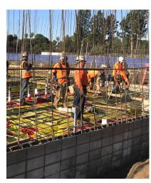
The masonry contractors are on site continuing to lay concrete blocks for the Stauffer gym. The underground utilities are complete, and the contractor is getting things ready for the concrete slab inside the building.
